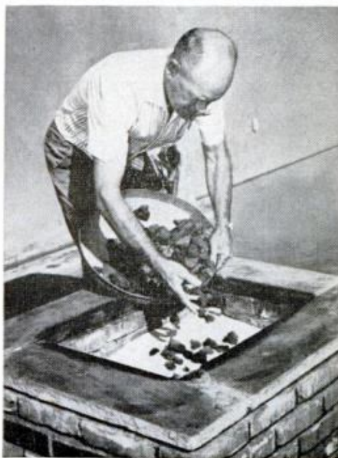
LAVA ROCK or cinders will catch some meat drippings, but both sand and rock must be replaced when grease accumulates
