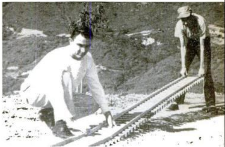
CLUB MEMBERS help install 1½-inch scale tracks at Johnson's mountaintop spread. Aluminum rails are held to redwood ties by miniature steel spikes
