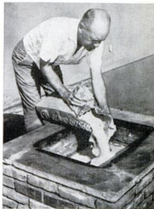
YOU CAN BUY white silica sand in 100-lb. sacks from almost any sand and gravel company. It holds and reflects the heat
