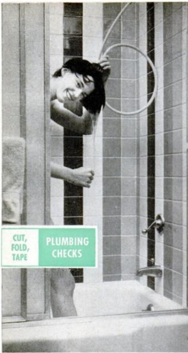
HOOKED TO A SHOWER HEAD , instead of a lavatory faucet, shampoo rinse hose is high enough so that its nozzle can't cross-connect with the water in tub
