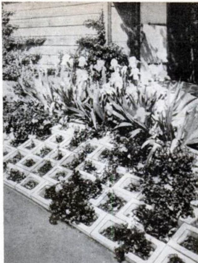
BLOCK GARDEN is a decorative solution to the problem of an eroding slope. Simply set tiers of single-core concrete blocks into the face of the slope, fill each core with top soil and plant as desired
